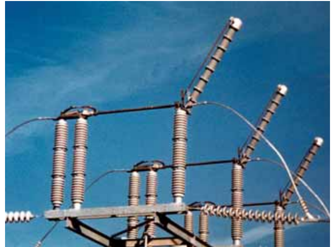
138kV typical full load-break switch combining the Series JMVI Interrupter with the Joslyn Hi-Voltage™ Series RF-2 Vertical-Break Switch. The Series JMVI Interrupter converts the isolating switch for full load switching at system voltages up to 230kV.
